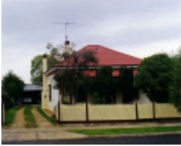
SL 122 - House, 13 Johnson Street, STAWELL
