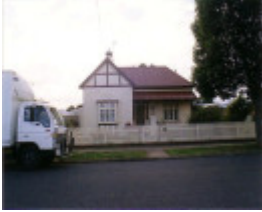
SL 124 - House, 3 Kofoed Street, STAWELL
