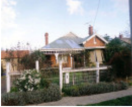
SL 126 - House, 6 Kofoed Street, STAWELL
