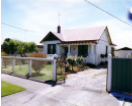
SL 128 - House, 15 Kofoed Street, STAWELL
