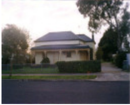
SL 130 - House, 23 Kofoed Street, STAWELL
