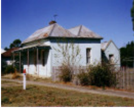
SL 132 - House, 5 Lake Road, STAWELL
