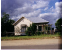
SL 135 - Former Telegraph Office, 21 Leslie Street, STAWELL
