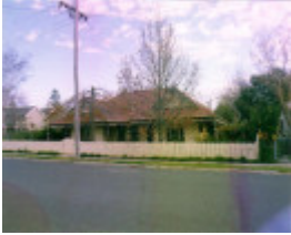
SL 142 - House, 'Terang', 33 Ligar Street, STAWELL
