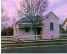
SL 149 - House, 58 Ligar Street, STAWELL
