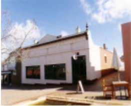
SL 164 - Stawell Club (former Star Hotel), 133-137 Main Street, STAWELL
