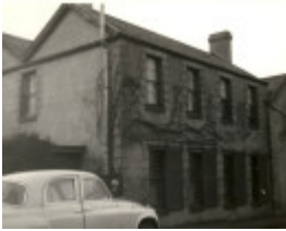
B1185 Former Knowle House
