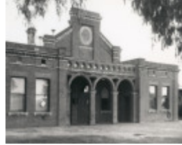
B2233 East Loddon Shire Hall
