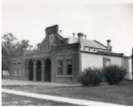
B2233 East Loddon Shire Hall
