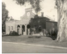
B2233 East Loddon Shire Hall
