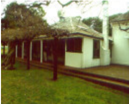
1 killeen homestead with verandah august2000.jpg
