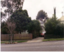
SL 171 - House, 15 Main Street, STAWELL
