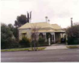
SL 172 - House, 17 Main Street, STAWELL
