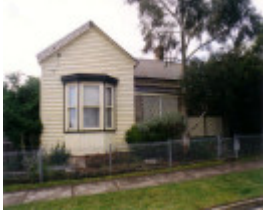
SL 175 - House, 27 Main Street, STAWELL
