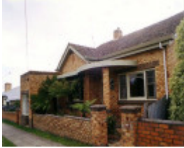
SL 177 - House and Shop, 39 Main Street, STAWELL
