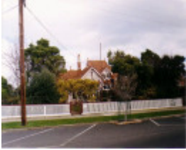
SL 178 - House, 40 Main Street, STAWELL
