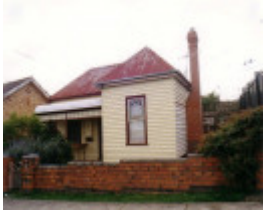
SL 179 - House, 41 Main Street, STAWELL
