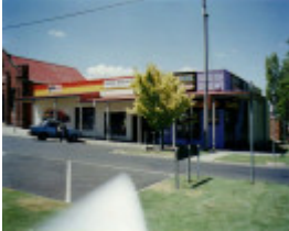
SL 181 - Shops, 46-48 Main Street, STAWELL
