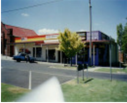
SL 181 - Shops, 46-48 Main Street, STAWELL
