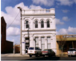
SL 184a - Former State Savings Bank, 60 Main Street, STAWELL
