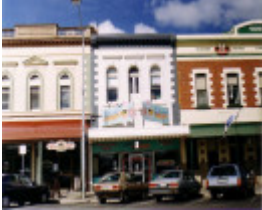
SL 186 - Shop, 70 Main Street, STAWELL
