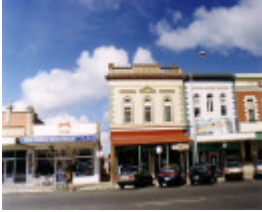
SL 187 - Shops. 72 Main Street, STAWELL
