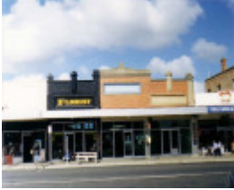
SL 188 - Shops. 78-82 Main Street, STAWELL
