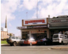
SL 189 - Shops, 'Stawell Taxis' & 'McDonalds Hairdressing', 79 Main Street, STAWELL
