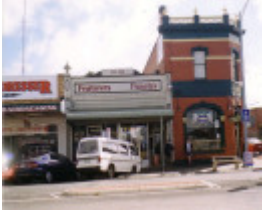
SL 190 - Shops. 81-83 Main Street, STAWELL
