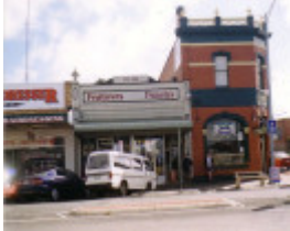
SL 190 - Shops. 81-83 Main Street, STAWELL
