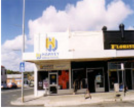
SL 191 - Shops, 84-86 Main Street, STAWELL
