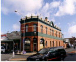
SL 192 - Two-storey building, 85 Main Street (corner Wimmera Street), STAWELL
