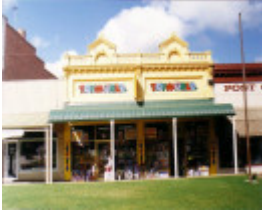
SL 195 - Shops, 90-92 Main Street, STAWELL
