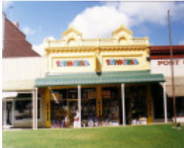
SL 195 - Shops, 90-92 Main Street, STAWELL
