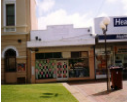
SL 196 - Shop, 91 Main Street, STAWELL
