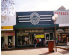
SL 198 - Shop, 97 Main Street, STAWELL
