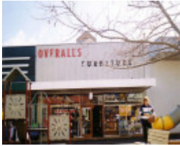
SL 199 - Shop - former Anthony and Co., 99 Main Street, STAWELL
