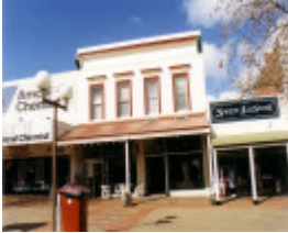
SL 200 - Two- storey Commercial Building, 100a Main Street STAWELL
