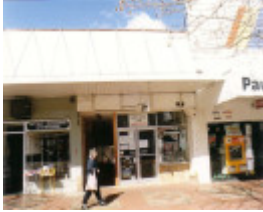
SL 203 - Shop, 108 Main Street, STAWELL
