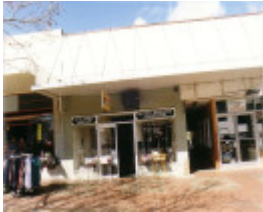
SL 205 - Shop, 110 Main Street, STAWELL
