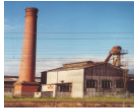
B6541 Former Australian Plaster Industries Boiler House
