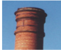
B6541 Former Australian Plaster Industries Chimney top
