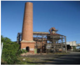
B6541 Former Australian Plaster Industries Boiler House
