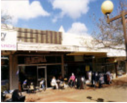
SL 207 - Shops, 112-114 Main Street, STAWELL
