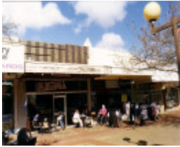
SL 207 - Shops, 112-114 Main Street, STAWELL
