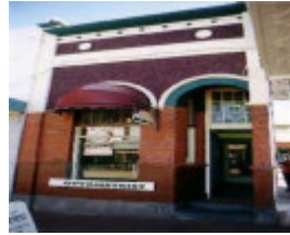
SL 210a - Shop, 119 Main Street, STAWELL
