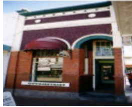
SL 210a - Shop, 119 Main Street, STAWELL
