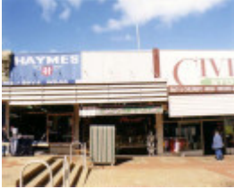
SL 211 - Shop, 120 Main Street, STAWELL
