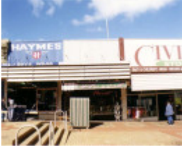
SL 211 - Shop, 120 Main Street, STAWELL
