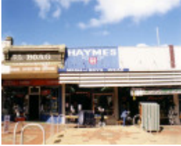
SL 213 - Shop, 122 Main Street, STAWELL
