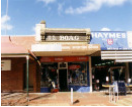
SL 214 - Shop, 124 Main Street, STAWELL
