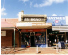
SL 214 - Shop, 124 Main Street, STAWELL
