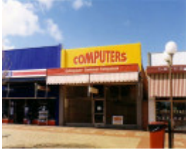
SL 220 - Shop, 'Grampians Personal Computers', 144 Main Street, STAWELL
