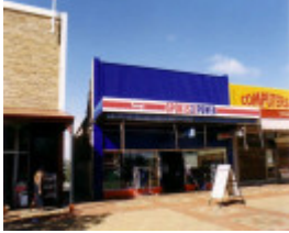
SL 221 - Shop, 146 Main Street, STAWELL
