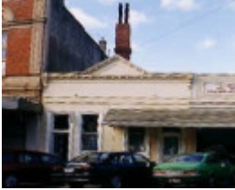
SL 228 - Shop, 164-166 Main Street, STAWELL
