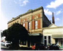
SL 230a - Former Free Library and Mechanics Institute, 168-172 Main Street, STAWELL
