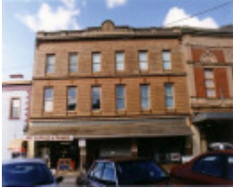
SL 233 - Former McKellar Building, 174-178 Main Street, STAWELL
