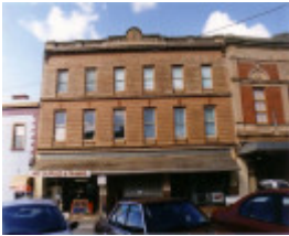
SL 233 - Former McKellar Building, 174-178 Main Street, STAWELL
