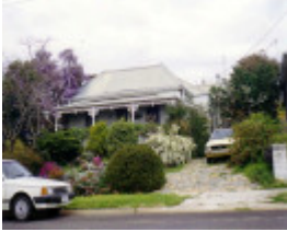
SL 235 - House, 226 Main Street, STAWELL
