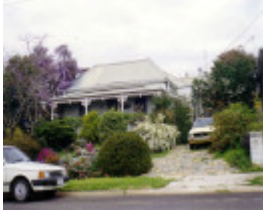
SL 235 - House, 226 Main Street, STAWELL
