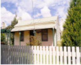
SL 244 - House, 24 Napier Street, STAWELL
