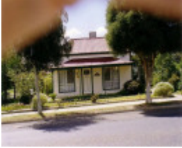
SL 245 - House, 29 Napier Street, STAWELL
