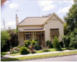
SL 246 - House, 31 Napier Street, STAWELL
